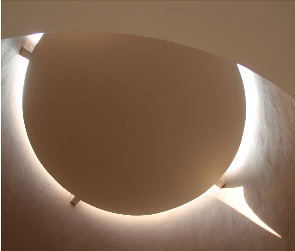
The skylight illuminating the undulating surface of the coarse mud rendered walls creates a dramatic sculptural element over the main seating of the living room.
